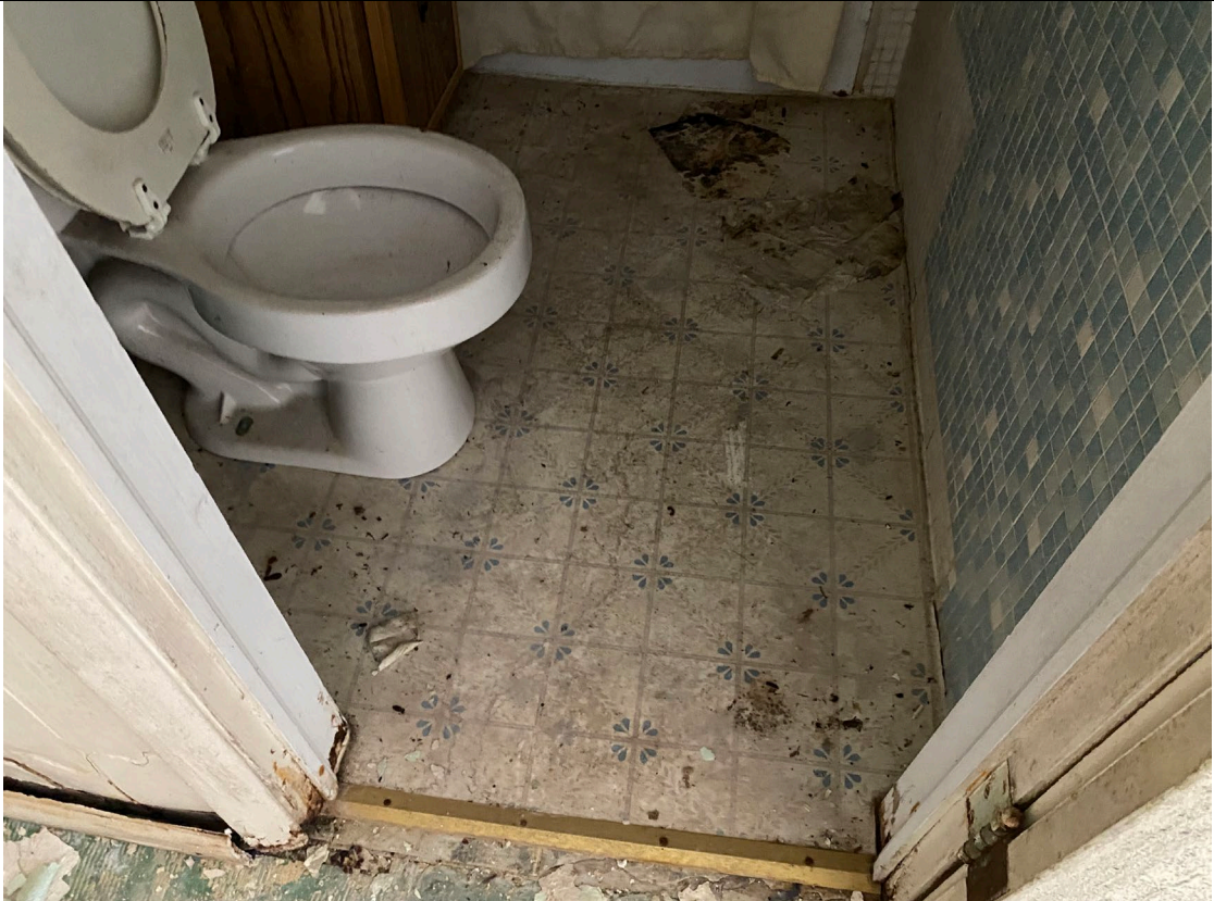
View of ACM Floor Tile in Restroom of Room 134
