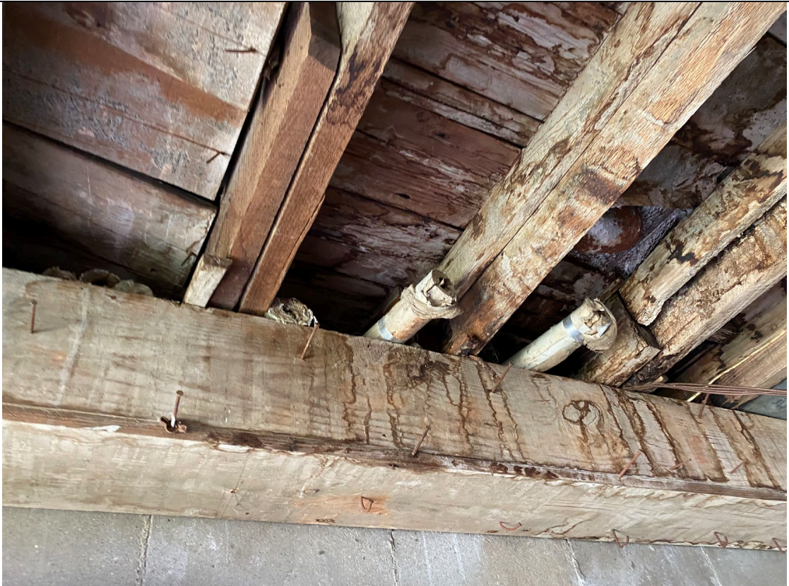
View of ACM Pipe Insulation
