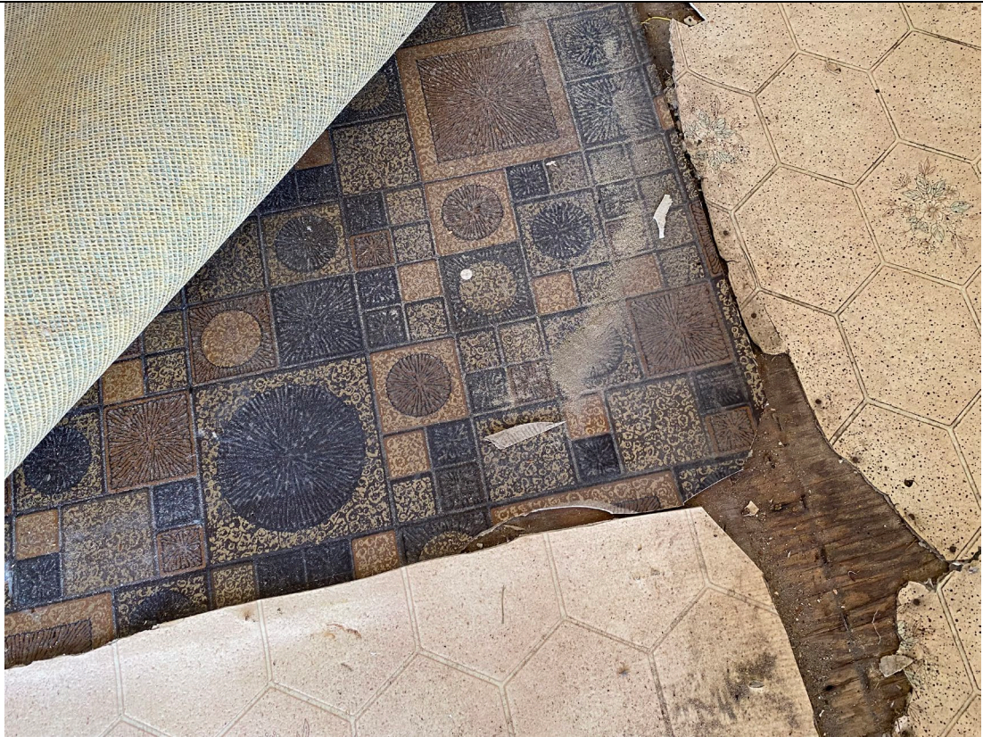
View of ACM Floor Sheeting in Office Storage Room
