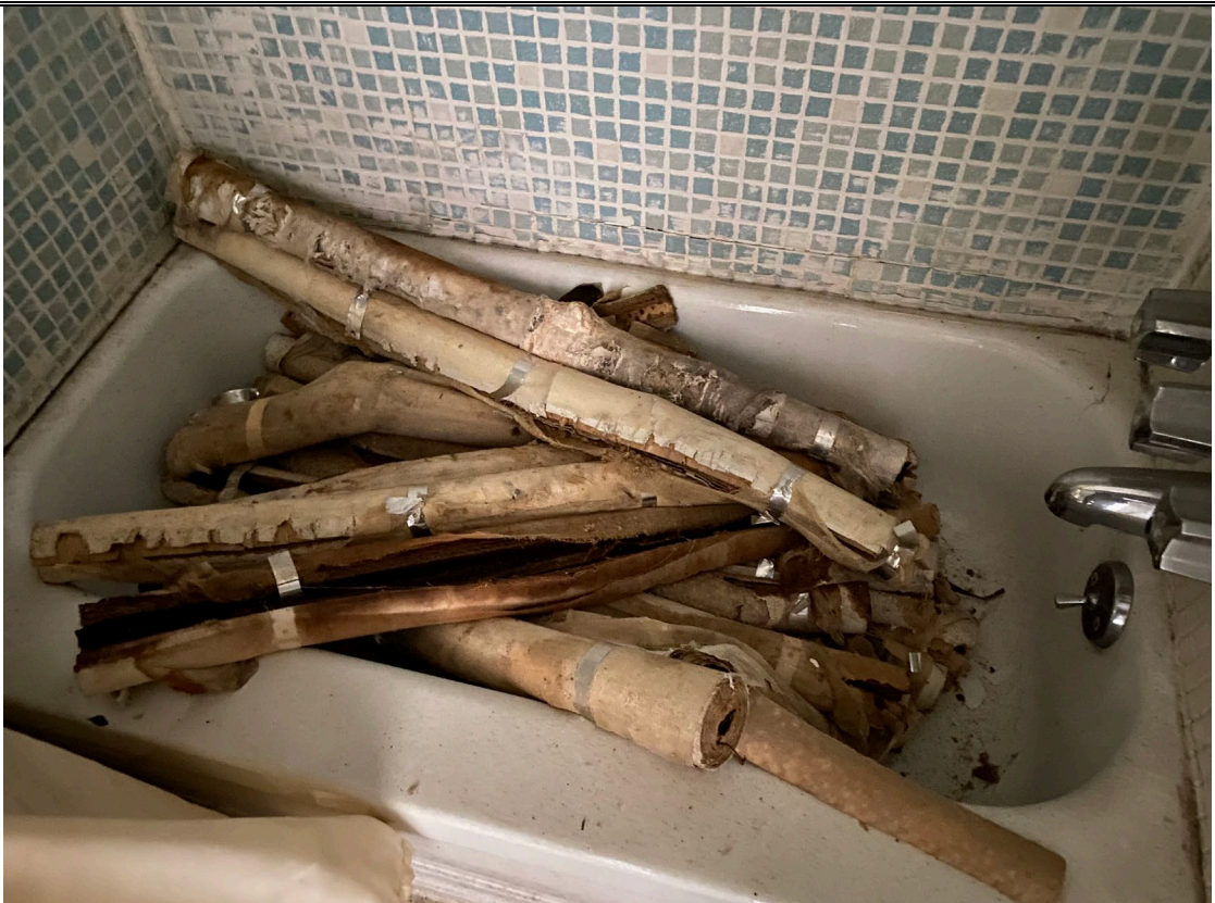
View of ACM Pipe Insulation as debris/garbage
